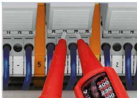
Function testing via touch-proof test slots.
