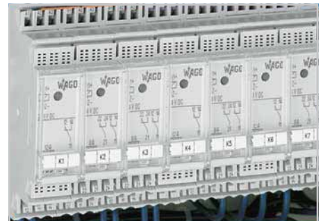
Marking via Mini-WSB Quick Marking System.
