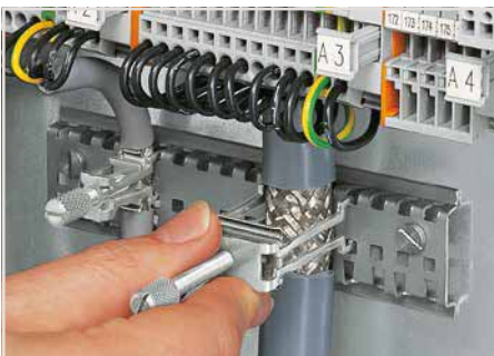
Fitting an additional clamping saddle.
