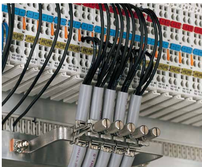
Figure 20: Application of the WAGO Shield Connecting System
