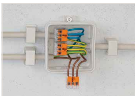
Wiring fine-stranded conductors in a junction box.
