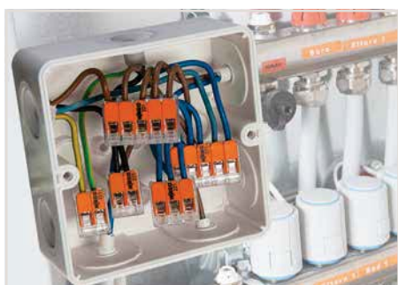
Wiring fine-stranded conductors in a junction box.
