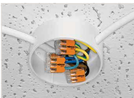
Lighting distribution in ceiling canopy
