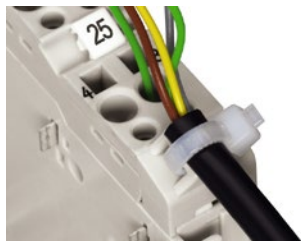
Figure 12: Attachment of Cable Binders
