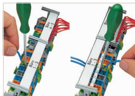
Sliding marking strips laterally.
